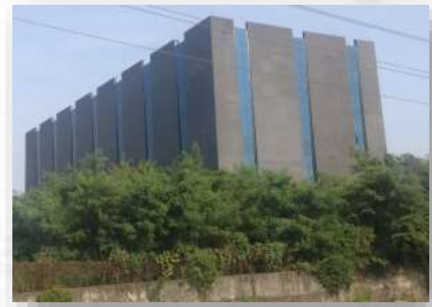
Control's Data Center, Mahape Midc
